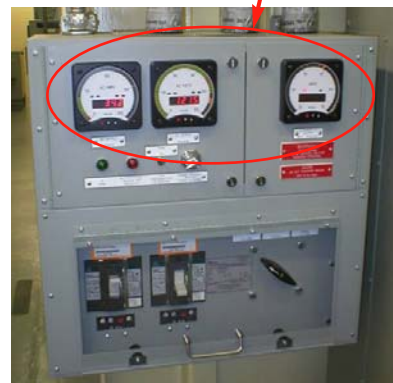
Power generation and distribution
