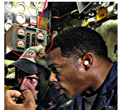
Engine room, loading bay & other local indicator panels
