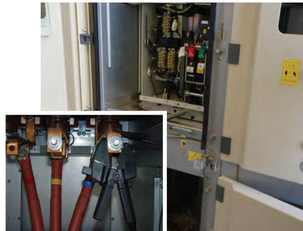
A new tough adjustable clamp has been designed to ensure flexibility in many applications and provides a good connection with the test piece
